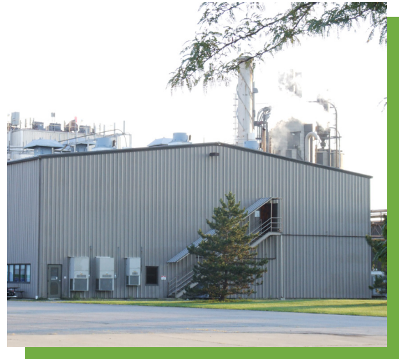
Sauder Co-Generation Plant
